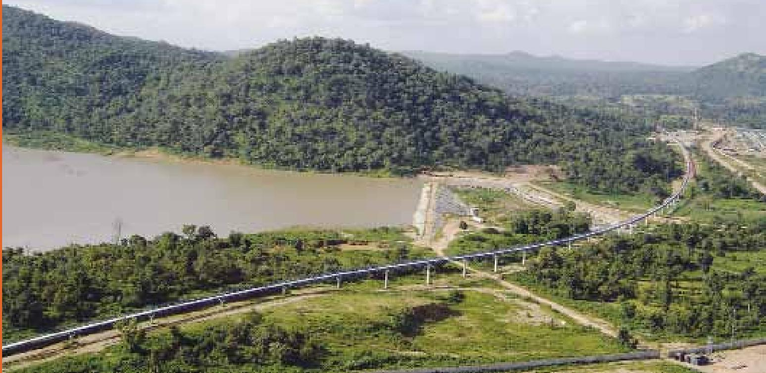
*The highly photogenic Obajana Cement conveyor in Nigeria. It is an elevated 7 km-long, 2 400 t/h conventional troughed conveyor – running at 5 m/s – in a triangular spaceframe support structure.*
